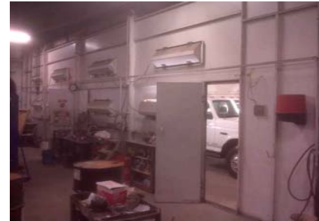
North Bldg - East Wall of Large Spray Booth
