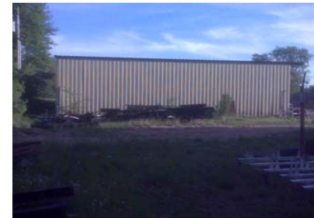
Main Bldg - View of North Side
