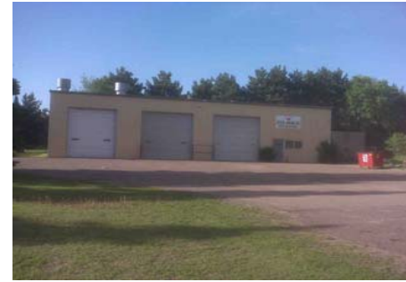
North Parts & Shop w/ Spray Booth
