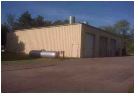
North Parts & Shop - Looking NE
